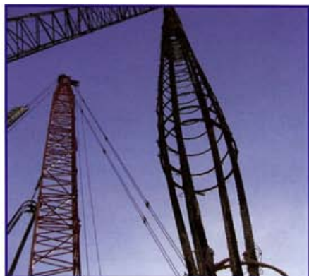
125 ft. (38m) of cage ready to place in grout
